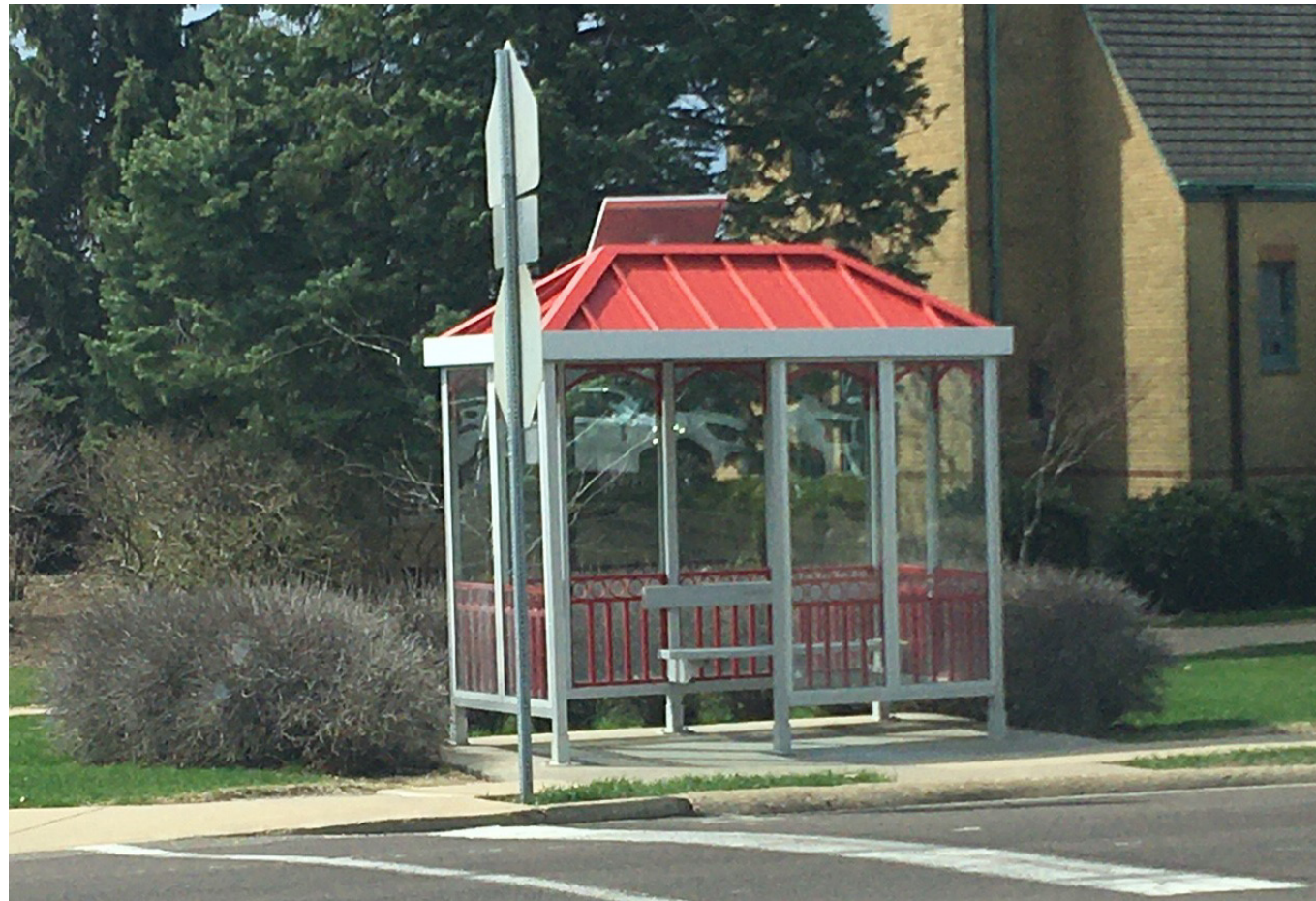
A major bus stop at Lake Avenue and Monroe Avenue with benches and proper ADA accessibility.
