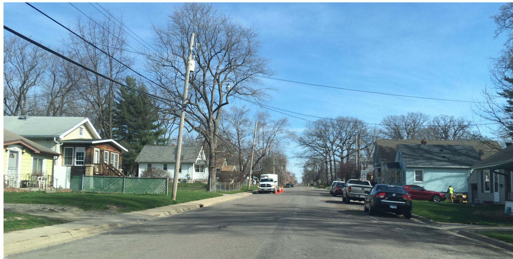
36' of pavement width within a 60' public right-of-way.
