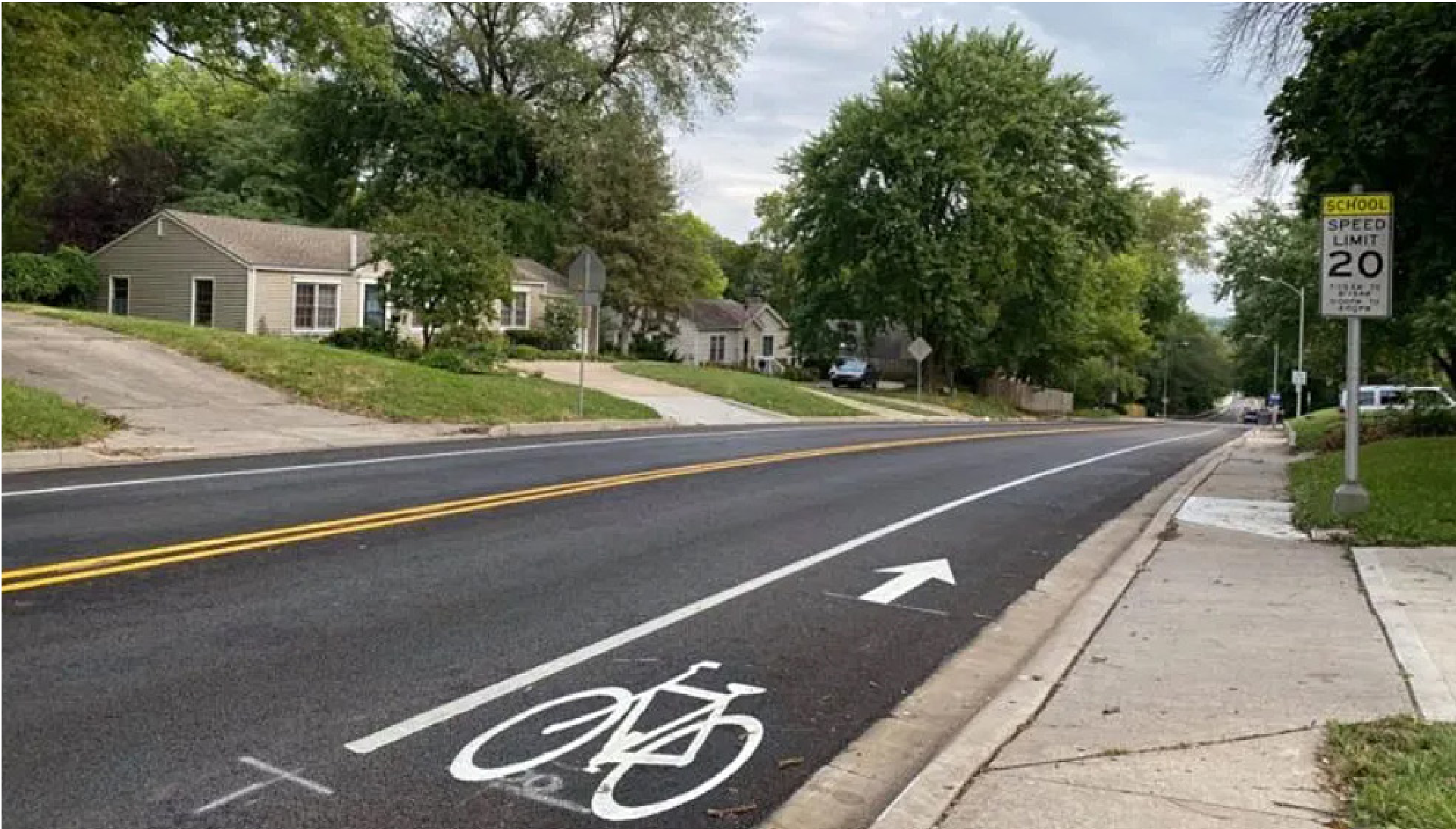
Dedicated bicycle lane adjacent to public sidewalk helps buffer pedestrians from vehicles.
